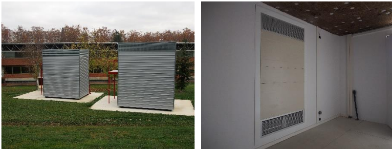
Figures 1 and 2: Integration of the Peltier Cells in façade (left) and interior view (right) of the thermoelectric prototype.
